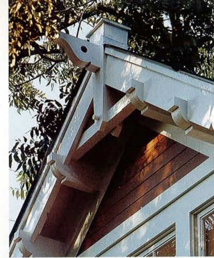
(CENTER) Wrapped by live oaks, this combination studio and garage becomes a backyard haven. Careful design and detailing help reduce the mass of the new two-story building. (LEFT) Timber brackets enrich the gable end above the studio's box bay.
