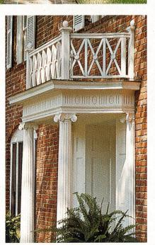
Richly detailed in the classical manner, the portico offers weather protection for guests. Stock Ionic columns support the roof structure; routed vertical grooves in the horizontal band replicate the triglyphs of ancient Greek architecture.
